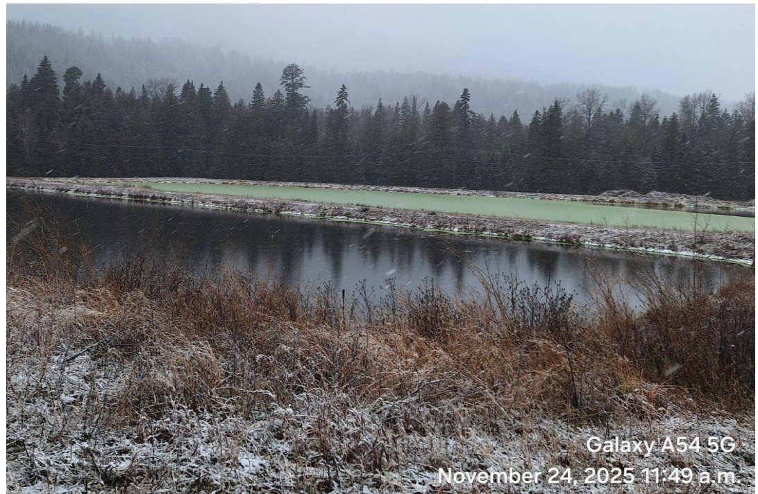
Photo 1: A view south-west of the Infiltration Basin #1 and the storage basin in the background at the City of Fernie's wastewater Facility.
